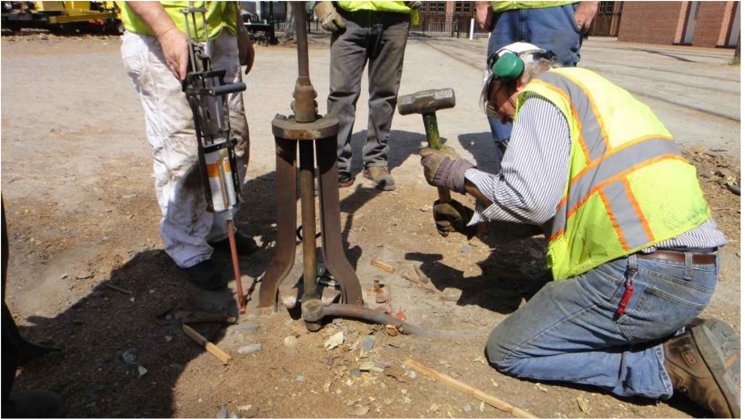
Steve N. employs his world-famous as-seen-on-TV windmill spiking technique with the short-handled sledge
