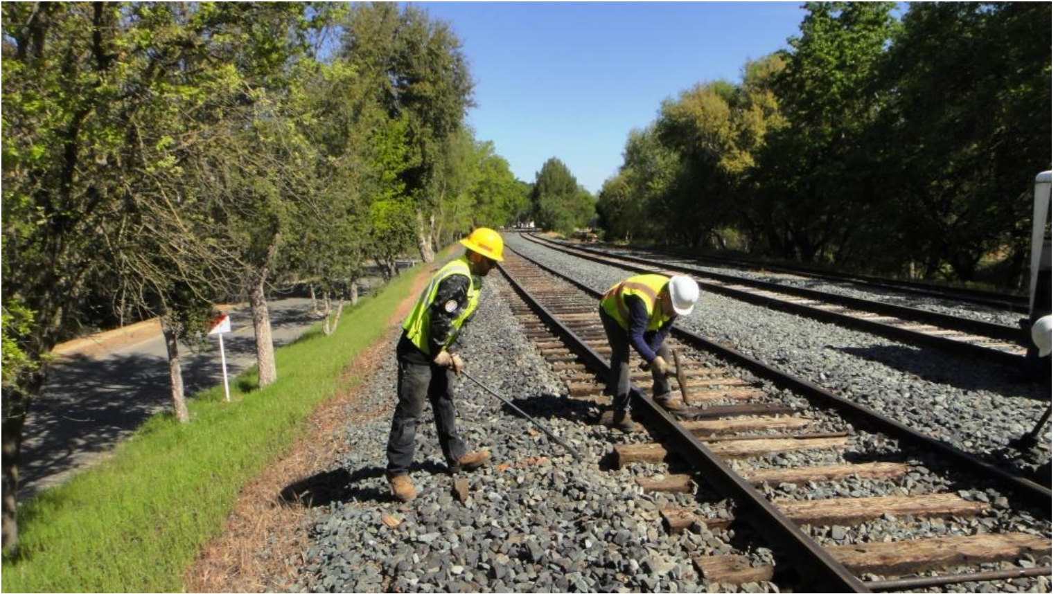
Chris and Steve W. nip and spike a previously un-spiked tie
