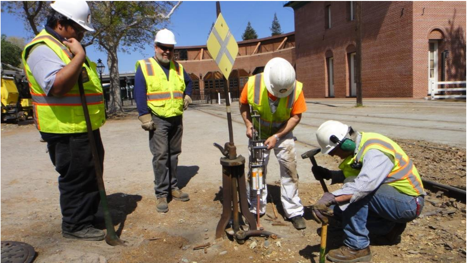
Mike H. injects a special epoxy-resin goo into the head-block to help stabilize it as Steve N. pounds in a tie-plug
