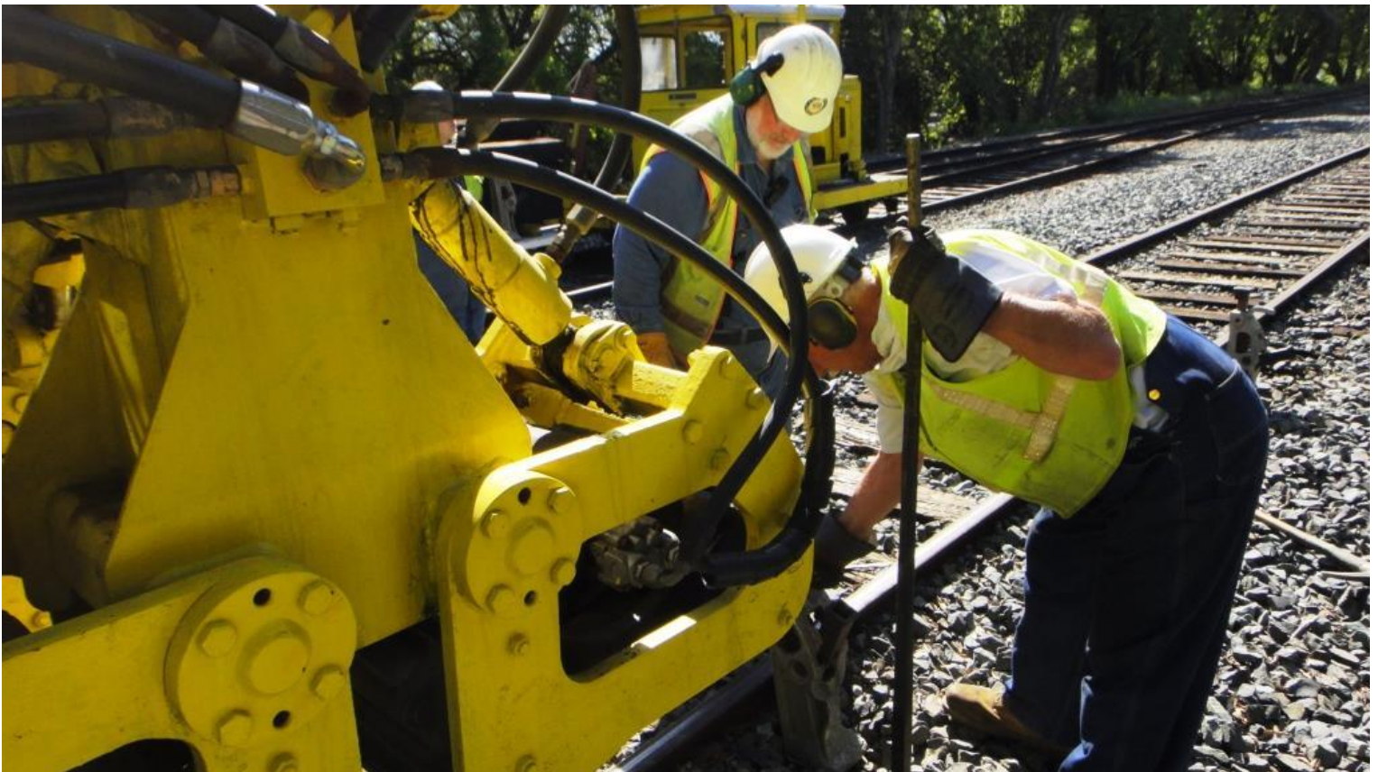
Clem and Frank remove a track-jack as the tamper approaches
