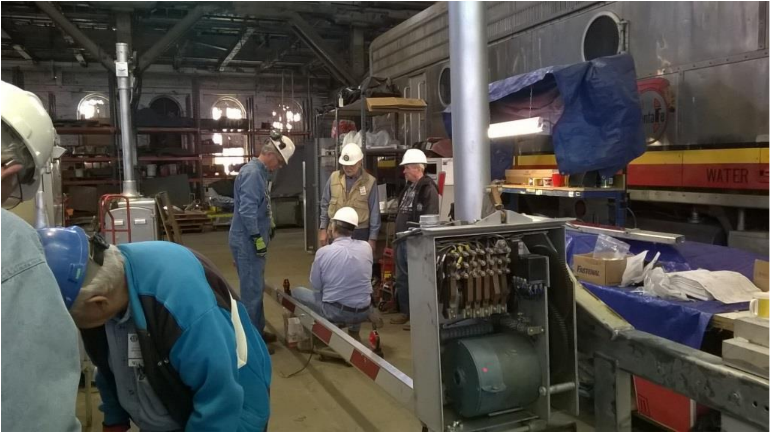
Team Signals working on building a whole new signal mast from scratch
