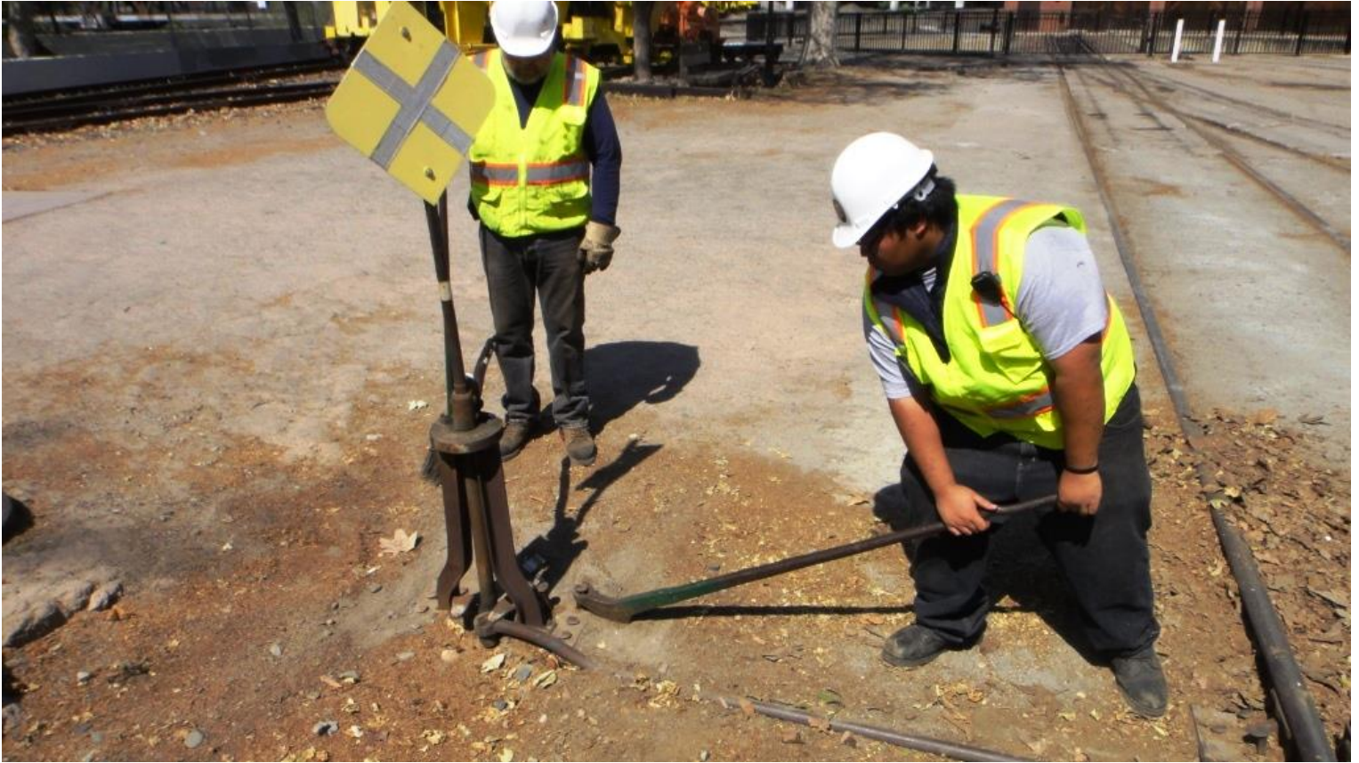
Anthony pulls spikes at Switch No. 2
