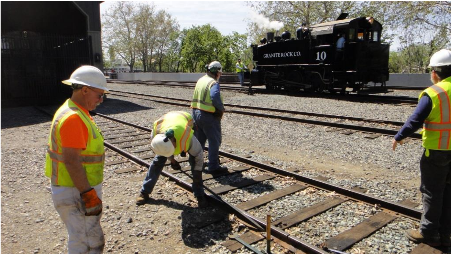
With bolts removed, Steve N. uses a lining bar to try to pry-off the broken joint-bar...
