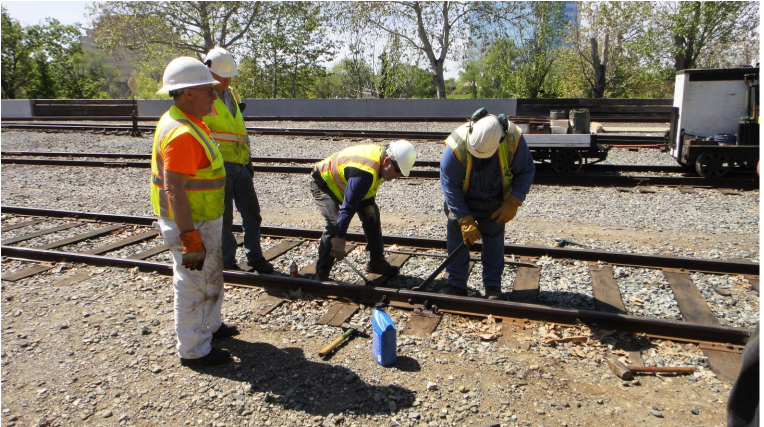
With the new joint-bar in place, Steve W. and Frank tighten-down the bolts
