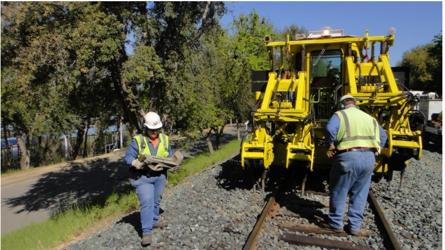
Heather removes a jack as Mike F. in the tamper continues tamping under Frank's guidance
