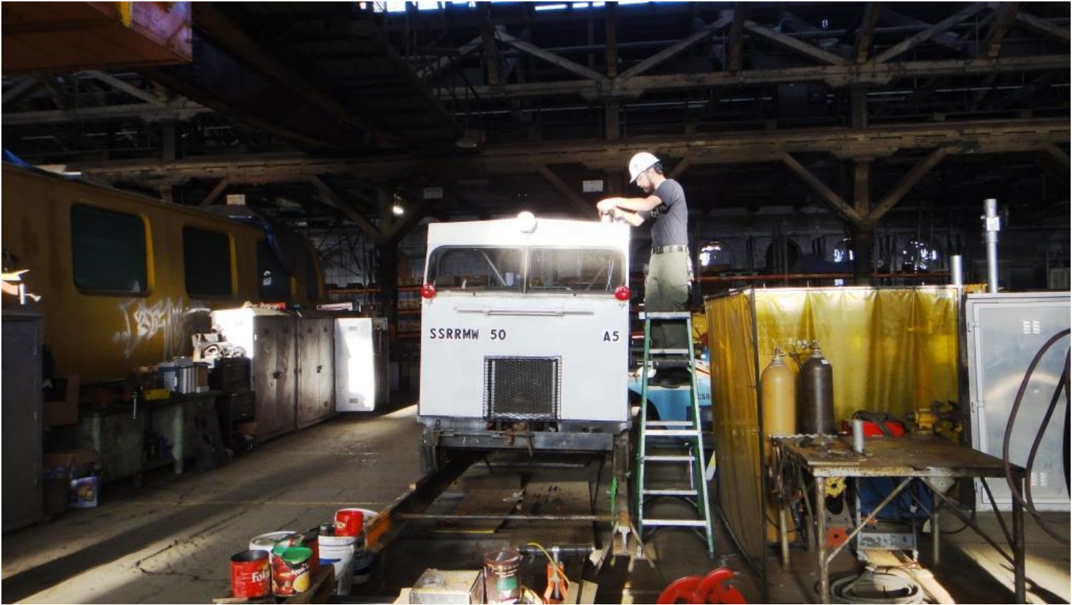
Matt installing new horns on the A-5
