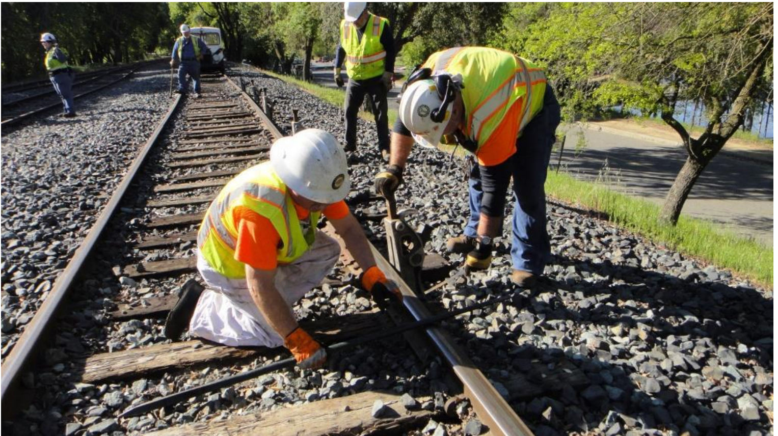
Mike H. and Mike F. use a special tool to remove debris from between a tie-plate and the tie to provide for a flush fitting
