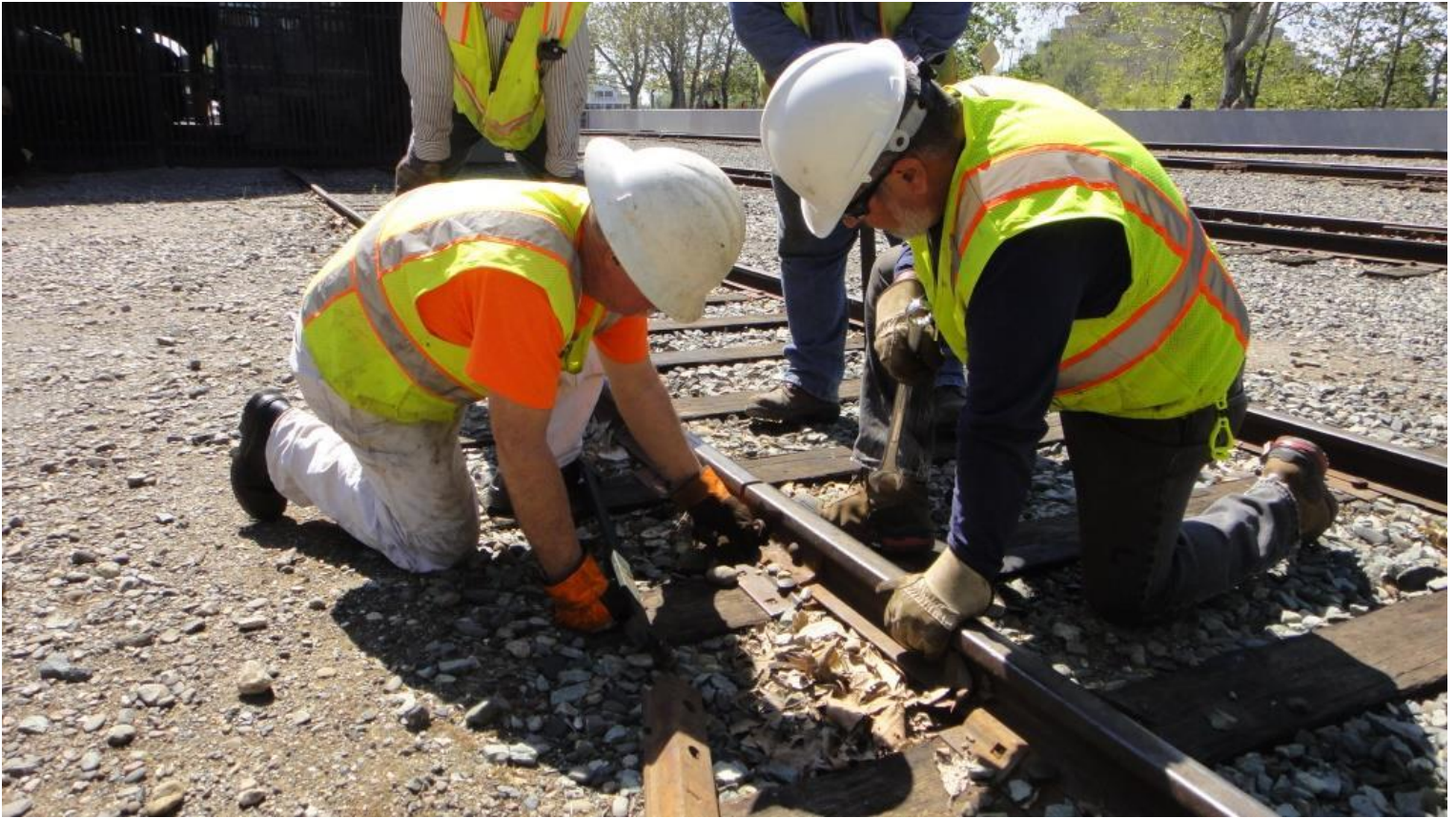
In Old Sacramento, Mike H. and Steve W. remove the bolts at the broken joint-bar
