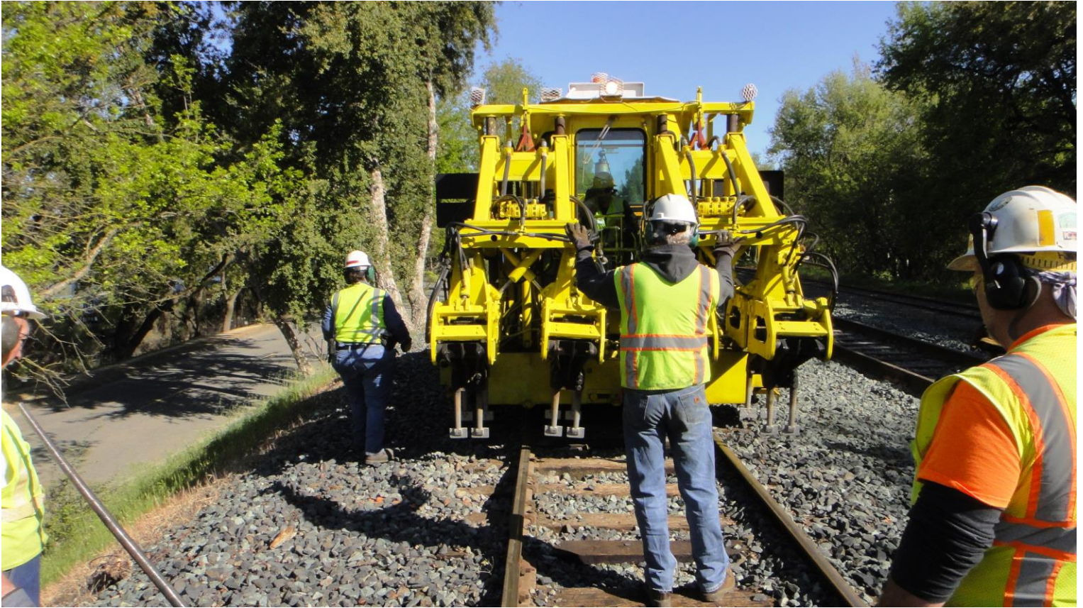
Steve N. guides Chris in the tamper as he tamps the rail to its new level
