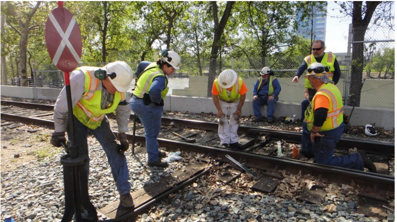
At Switch 101, the Team works resolve the difficulty to throw problem
