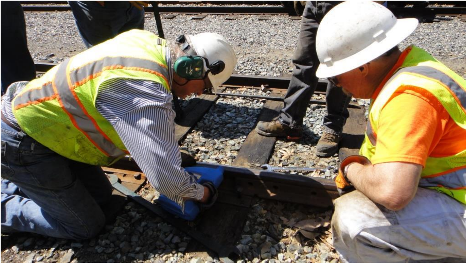
Steve N. applies a little oil behind the joint bar to help with thermal expansion
