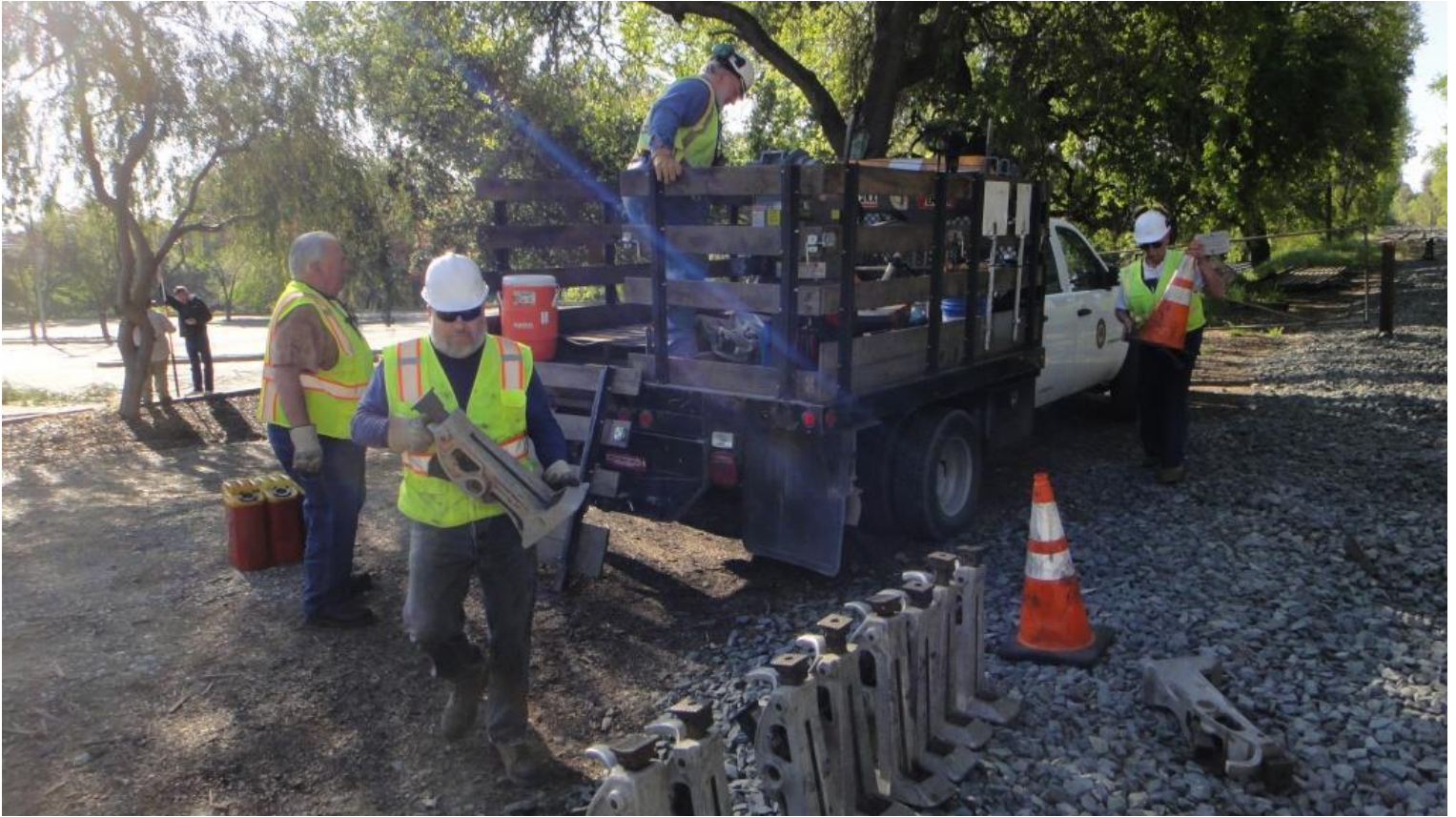
Steve W. unloads track-jacks from the back of the truck
